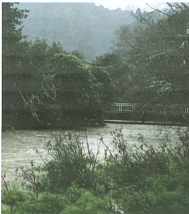
#5B - Brook Stream - close up of the flood running under the Domett St bridge - with only around 15 cm of clearance
