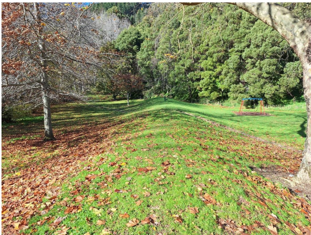
Photograph B.1: Stopbank within Hanby Park on the true left side of the Maitai River.
