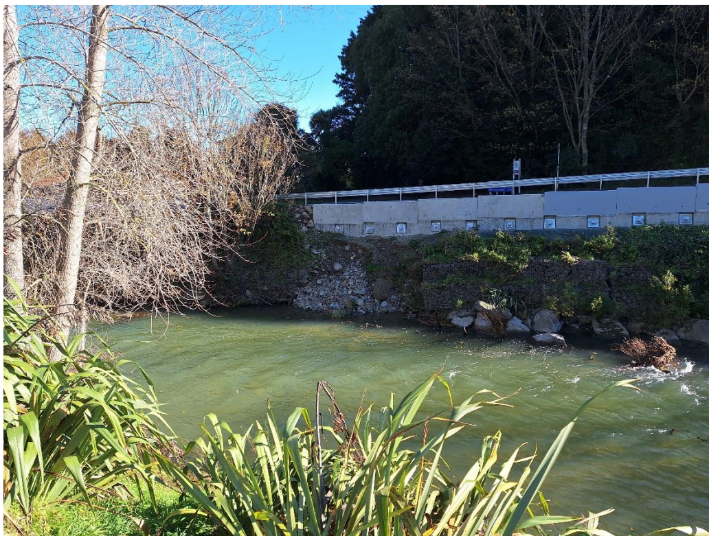
Photograph B.11: The true right banks of the Maitai river and the barriers of Matai Road. A previous slip is evident and gabion baskets as scour protection can be observed.
