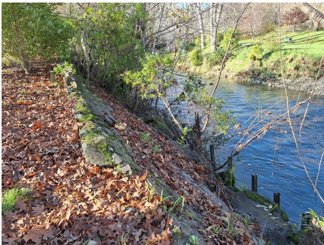
Photograph B.16: Rammed railway irons line the river bank as scour protection.
