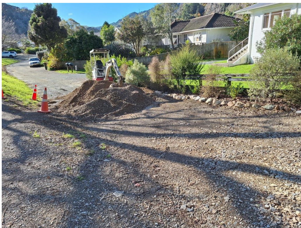
Photograph B.8: On the road at the end of Clouston Terrace is a pile of gravel (6m x 3m) with a small excavator sitting on top of the pile.
