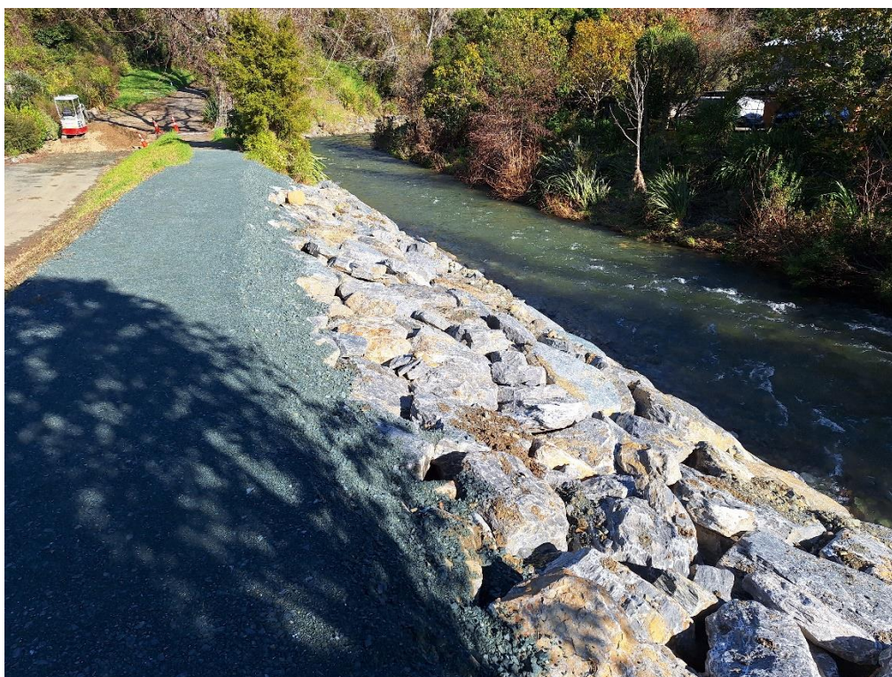
Photograph B.6: Recently laid gravel on the gravel path which runs along the top of the stopbank of the true left side of the river. Boulder protection can be observed on the river bank.
