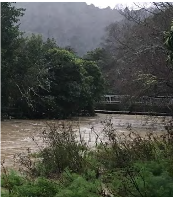
#5B - Brook Stream - close up of the flood running under the Domett St bridge - with only around 15 cm of clearance . The height of the underside of the bridge is just under 8 m from Nelson datum.
