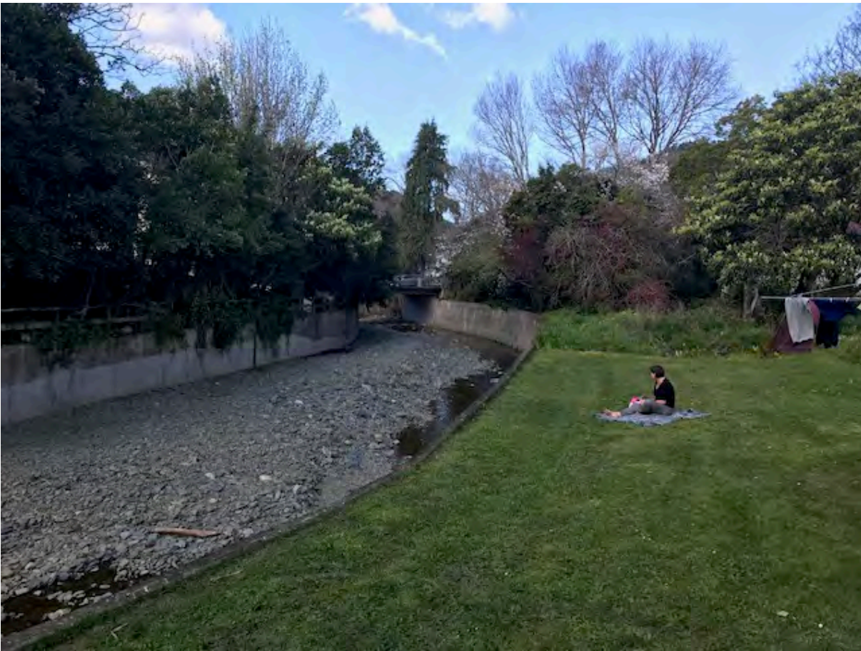
#4A - Brook Stream - looking down to Domett St bridge - normal flow
