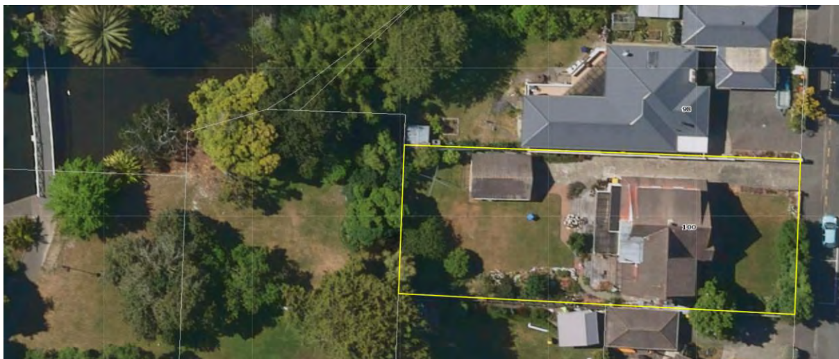
Figure 1 – 100 Tasman St (outlined in yellow) showing western shared boundary with the Queens Gardens.
