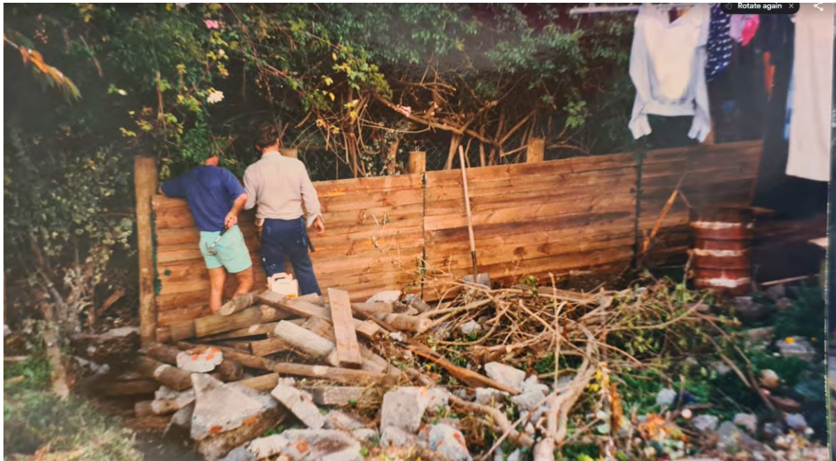
Photograph 1 – Retaining wall under construction. Note the base of the retaining wall is at the current ground level of the Queens Gardens.
