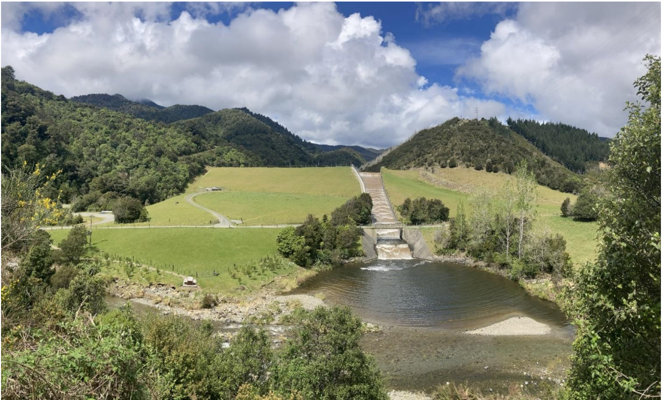
Maitai Dam spillway
