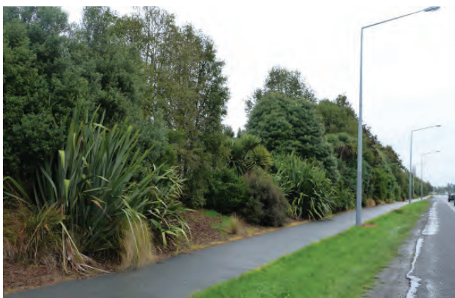
FIGURE 6 Noise and air pollution buffer separating residential property and Queen Elizabeth II Expressway, Northwest Christchurch with high biodiversity corridor values. This is a combination of a 3m high earth embankment (main noise barrier) planted with forest species to muffle the noise: Plagianthus (lowland ribbonwood/mānatu), pittosporums (kōhūhū and lemonwood/tarata), coprosmas (karamū and mikimiki), Griselinia (broadleaf/kāpuka), Cordyline (cabbage tree/tī kōuka), Dodonaea (akeake), Sophora (kōwhai), Phormium (NZ flax/harakeke), Pseudopanax (five-finger/whauwhaupaku), olearias and Hebe (koromiko) and Anemanthele (wind grass).
