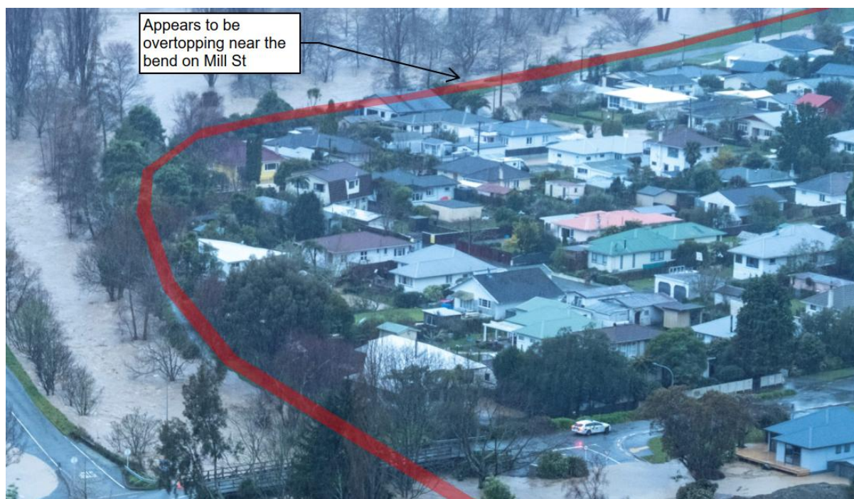
Figure 3.3: Flooding during the August 2022 storm. Time of photograph unknown.
