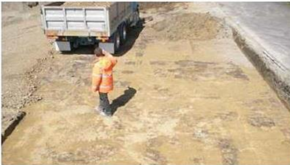
Pile holes and drains, house site
