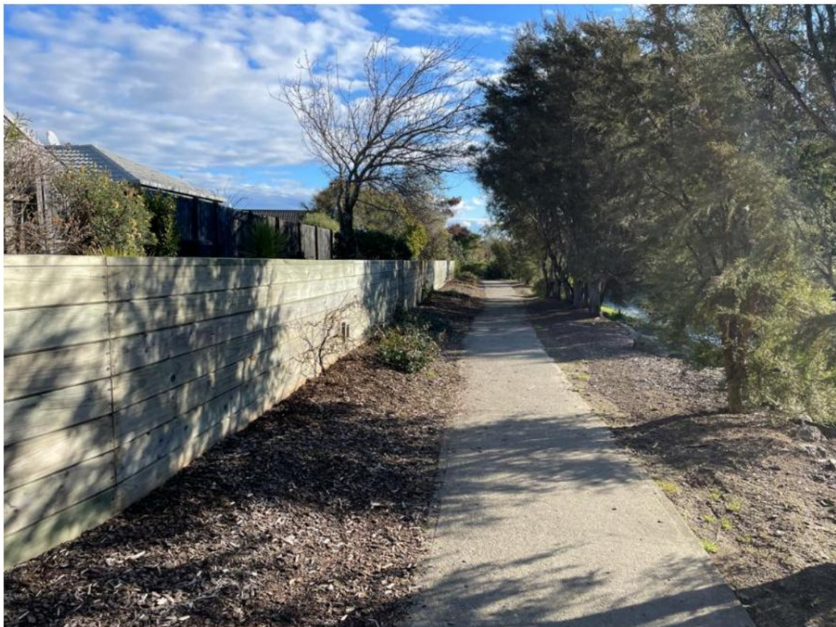
Figure 3.3: A photograph of a pole flood wall from another site in the Nelson region. This wall is similar in height to the proposed Portion 2 floodwall. (Source: Design Report, Appendix H)
