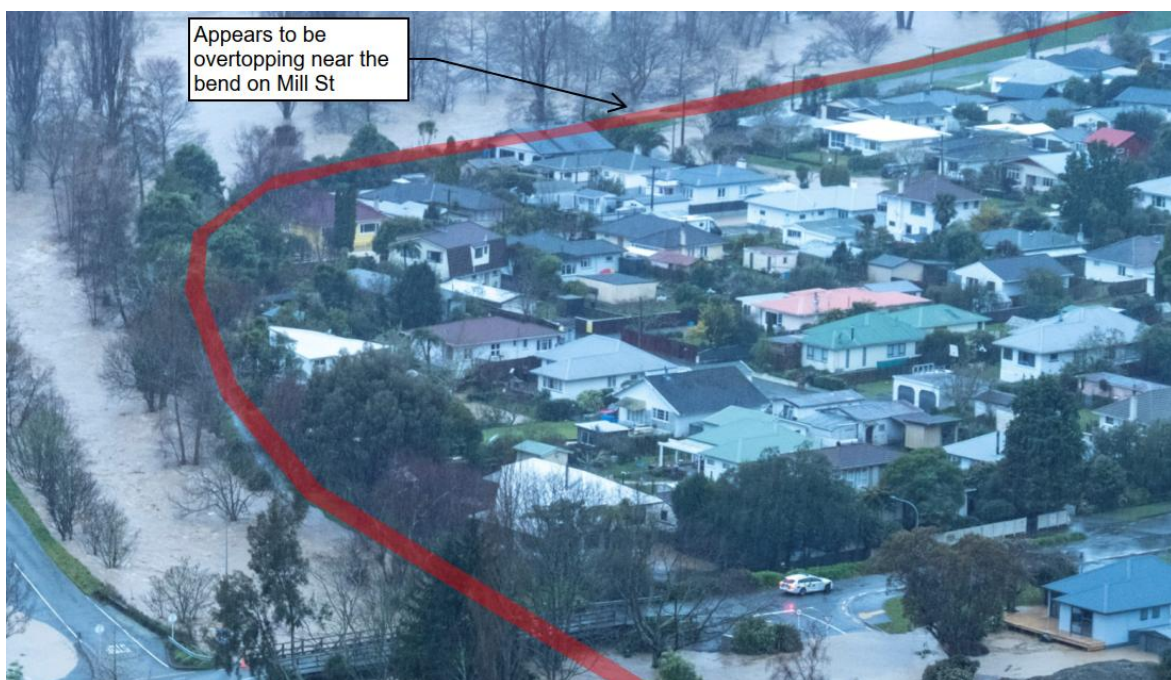
Figure 2.3 Photo showing extent of flooding across the Site during August 2022 flood event (red line indicates the existing stopbank between Clouston Bridge (foreground) and Hanby Park).
